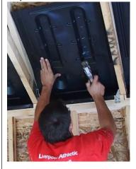
**Step 3:** Fully secure the ventilation baffle to the roof decking.
